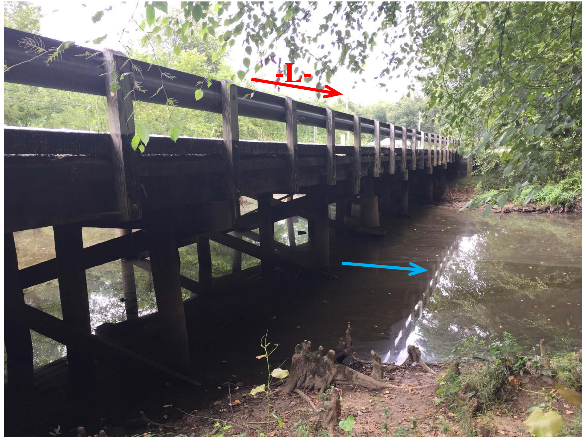
Looking East towards End Bent 2
